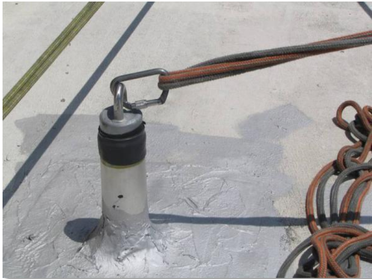
Roof anchors
