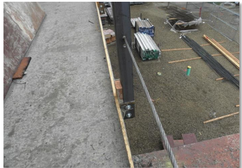
Panel and guardrail anchor points
