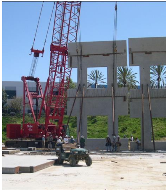
Concrete wall panels
