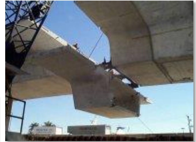
Concrete segmented bridge
