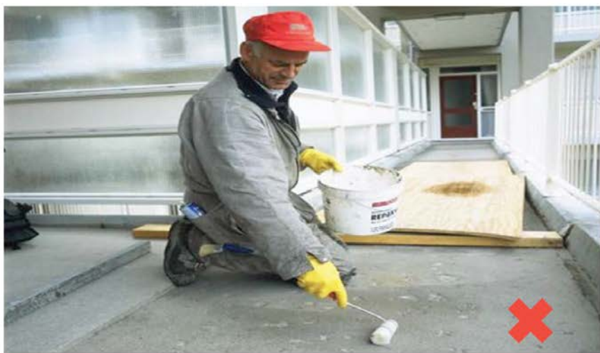
Figure 6 A floor coating being applied by a worker who is kneeling down and using a short-handled spreader
