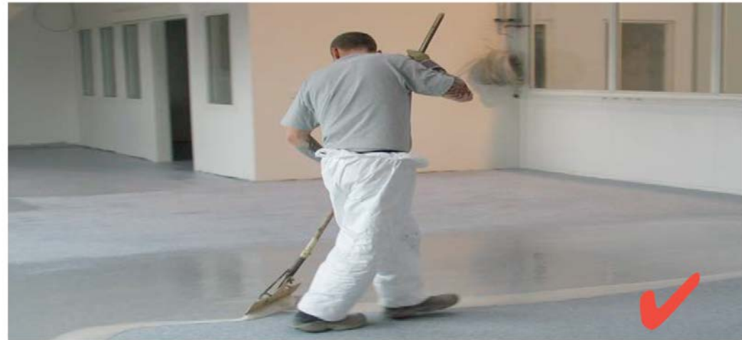
Figure 7 With the help of a long-handled spreader, an adequate safe working distance has been applied, reducing the likelihood of contact with the coating. It reduces the potential for back problems too
