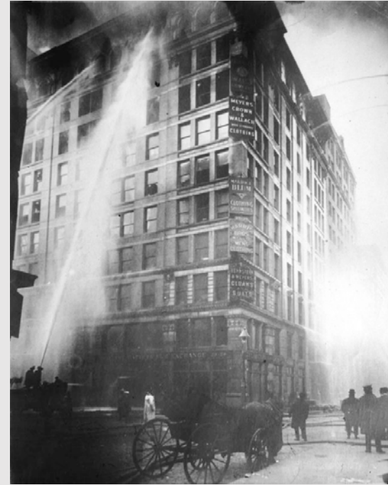
Presently the “Brown Building” 23-29 Washington Place, NYC
